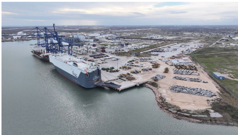
PHOTO CUTLINE: Aerial view of Velasco Terminal at Port Freeport, where 10 acres will be improved to enhance cargo handling operations.
